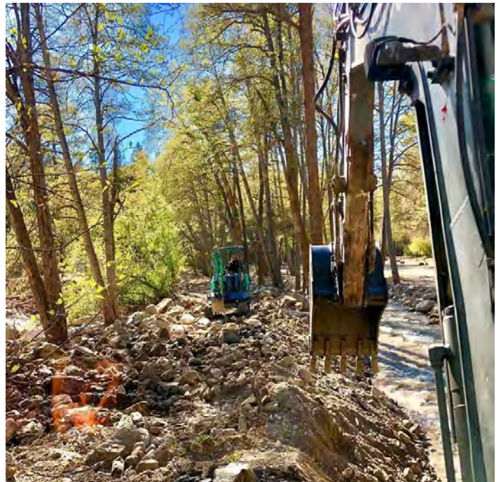
KT Enterprises Rebuilding the Seven-Oaks Resort
